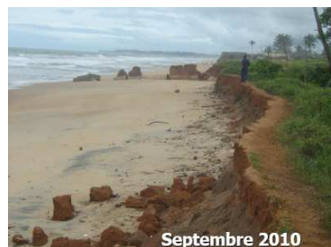
Figure 3: Coastal erosion at San Pedro (source: S. Yao).
