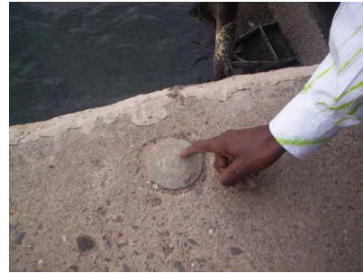
Figure 5: A location of the bench mark near the tide gauge station
