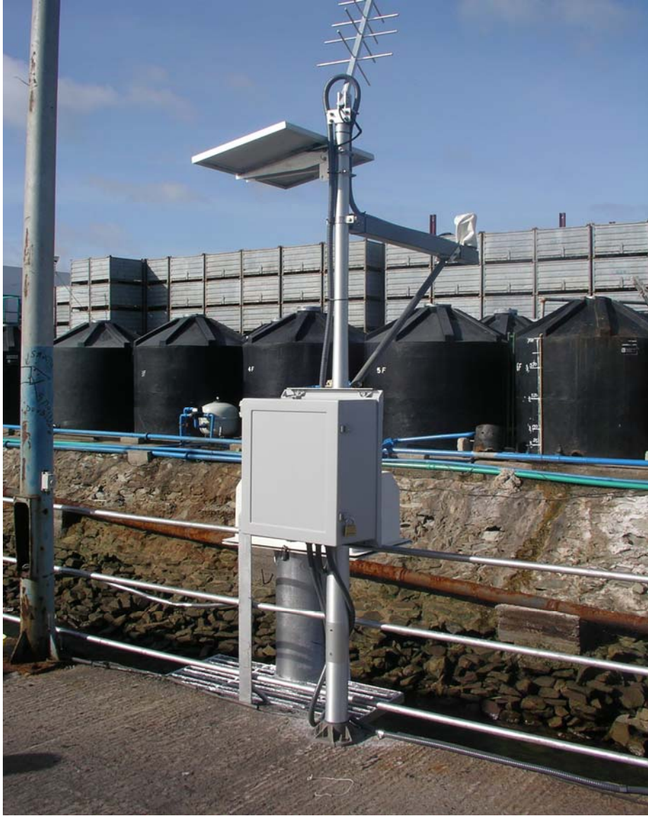
Photograph of Upgraded Mombasa Tide gauge
