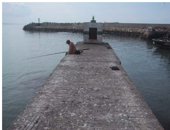
Figure 11, Essaouira Harbour entrance eastern jetty with electrical power available at the navigation light. Potential location for a radar tide gauge.
