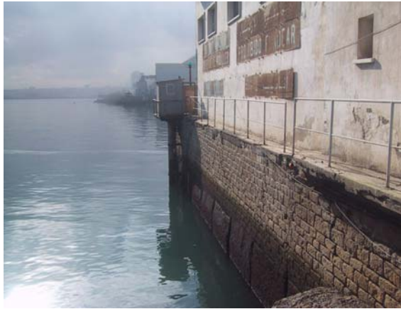
Figure 12, Casablanca Port Control Tower and old Tide Gauge alongside
