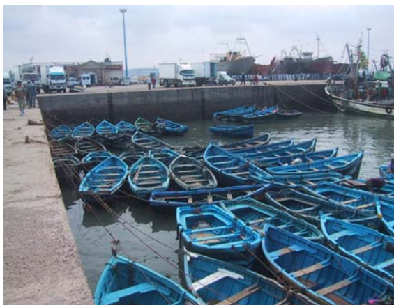
Figure 10, Essaouira. Inner Port Basin and fishing boats. Potential location for a stilling well/pressure sensor TG with secure cabinet & stilling well. Note: problems of fishing boats/mooring lines.
