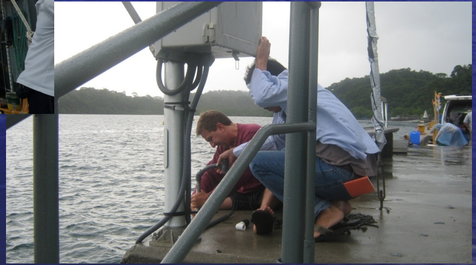
Installation of tide gauge equipment
