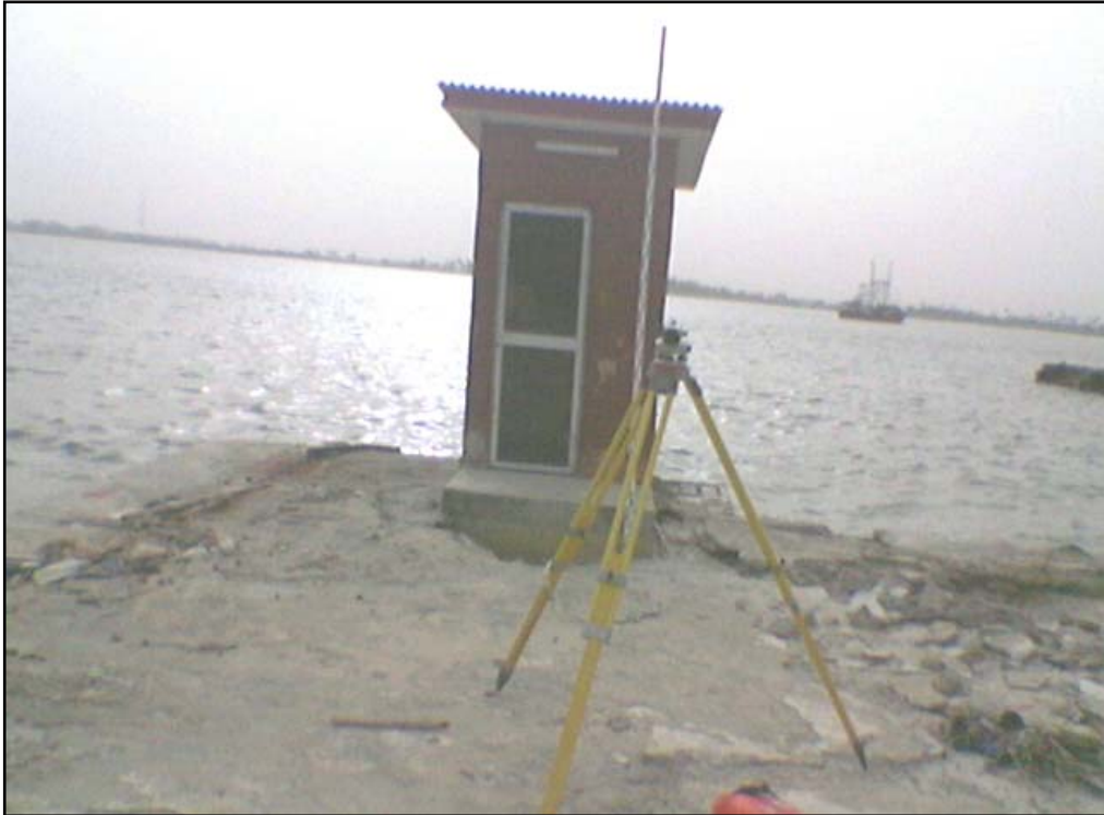
Figure 4. Newly constructed Kalestro tide gauge house at NIOMR jetty Lagos. (Entire Jetty is still awaiting rehabilitation)
