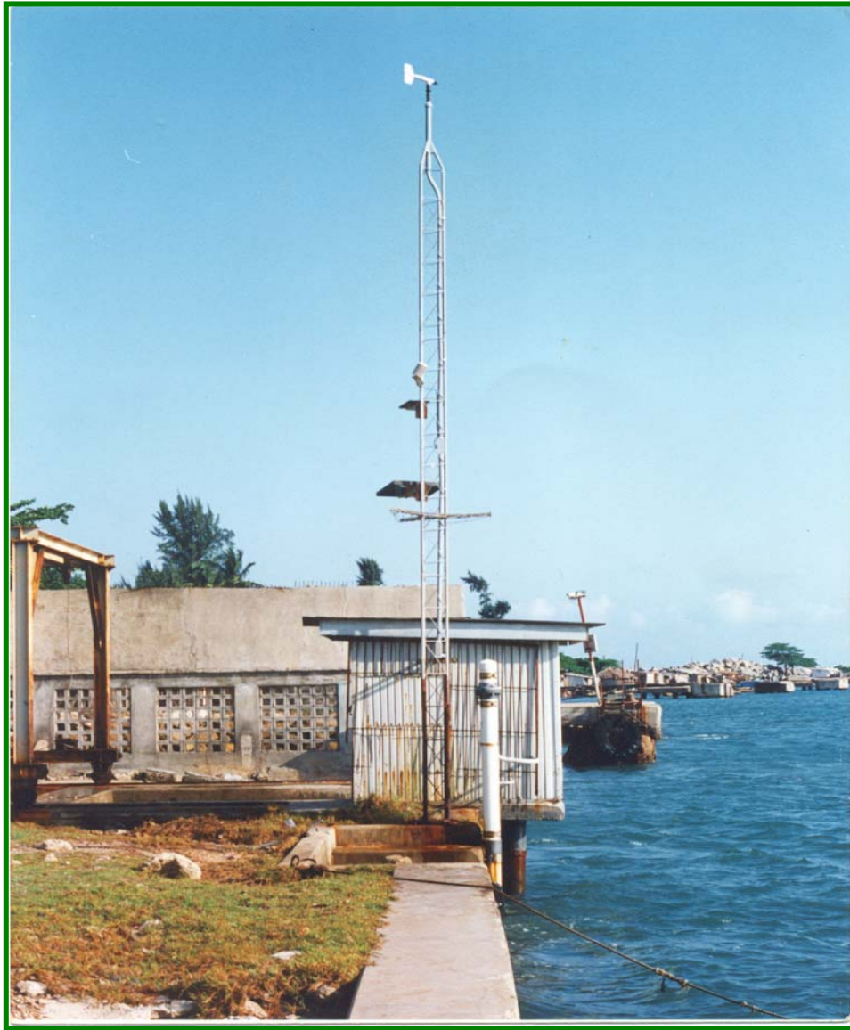
Figure 2. Picture of the Next Generation Water Level Measuring System (NGWLMS) installed at the NIOMR Jetty in the Commodore Channel Lagos before it was washed away during a storm in July 2000. (NGWLMS stilling well in white, analogue tide gauge stilling well in black under the housing, meteorological mast. NGWLMS computer and data logger inside housing).
