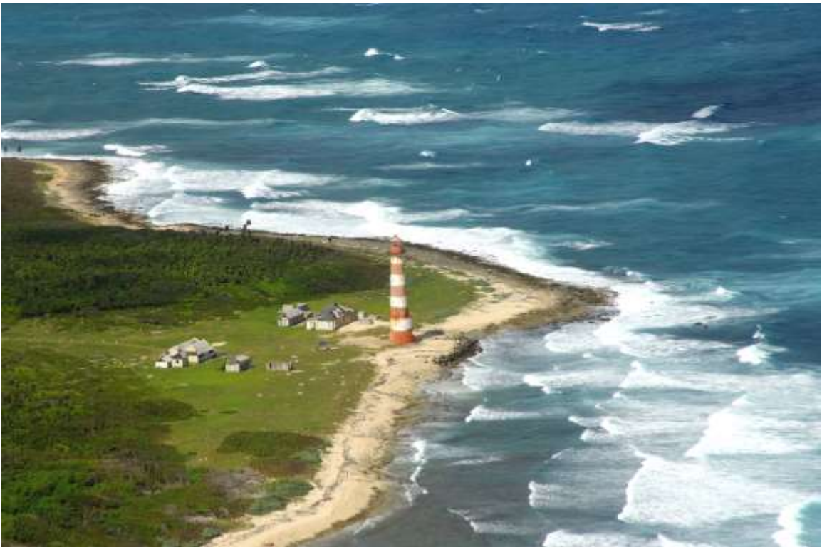
Morant Point Lighthouse, projected site of new Tide Gauge Installation
