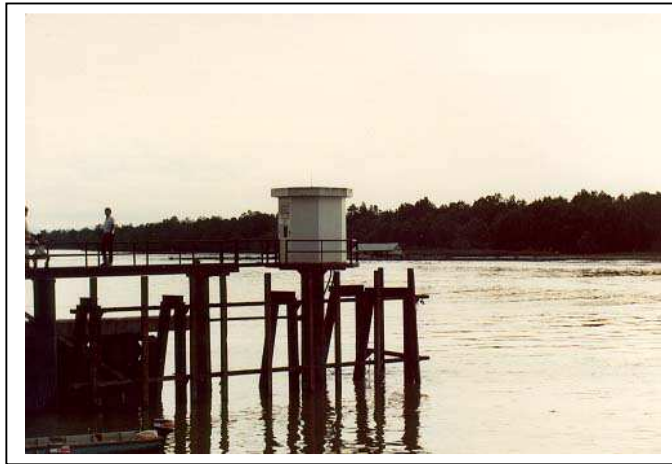
Example of a Tide Station
