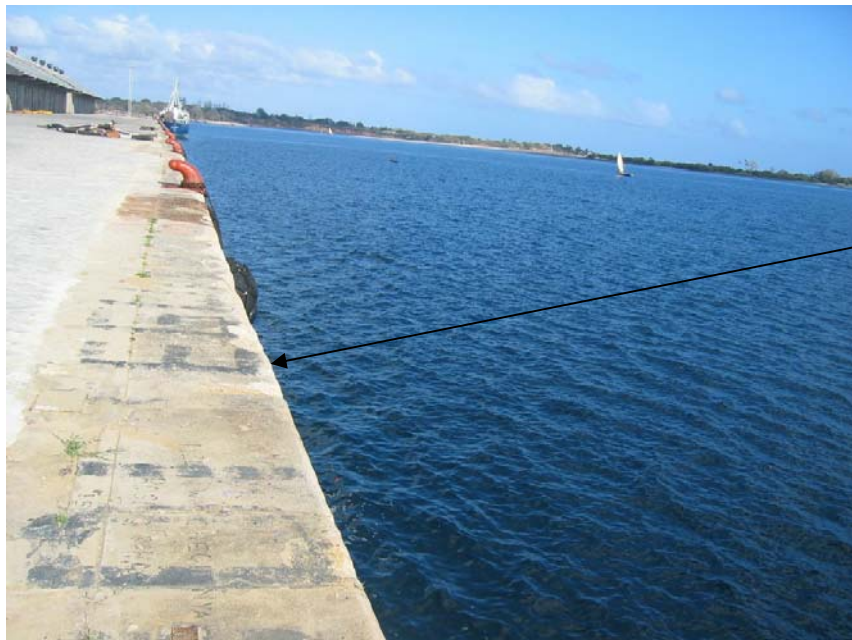
Figure 7: The arrow shows Mtrwara Port main quay
