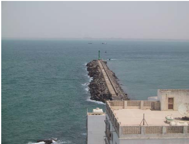
Fig 1. Ras Marbut Breakwater from the Port Control Tower. The CAMA tide gauge pressure sensor is next to the light tower at the end of the Breakwater.
