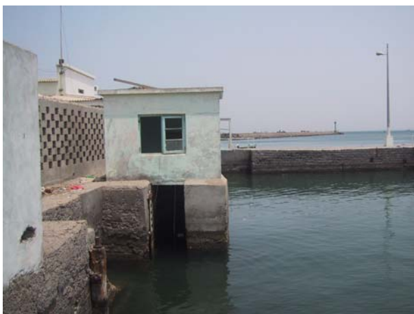
Fig 4. Pilots Pier Tide Gauge Hut housing the WS Ocean System SLM-2 Tide Monitor pressure sensor /stilling well, with Ras Marbut breakwater and Pilots Pier
