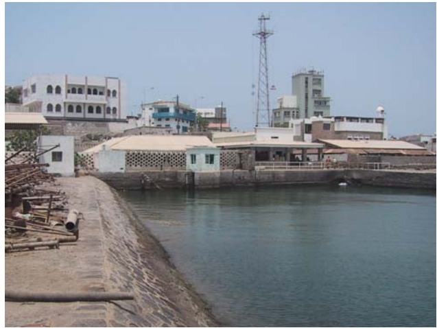
Fig 2. Port Control Tower, Tide Gauge hut (centre) and data logger hut (left of photo) with Pilots Pier on the right at Tawahi.
